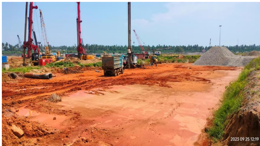
Ground Improvement (stone column erection in progress)
