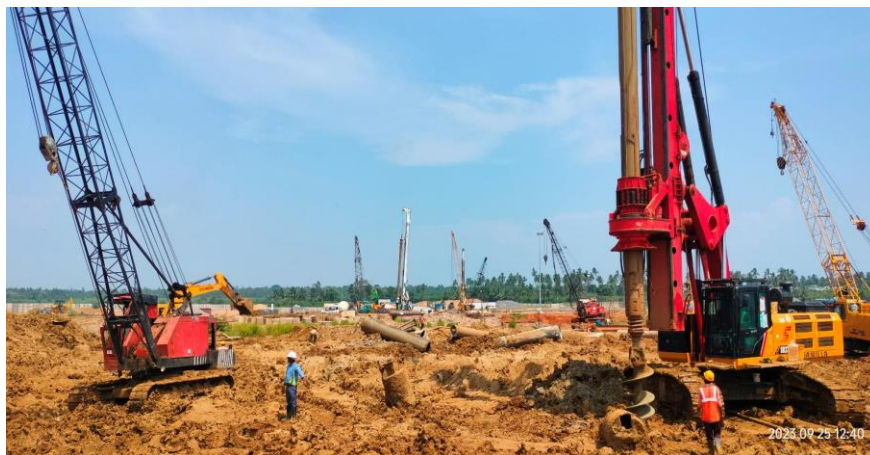
Piling work (in progress)
