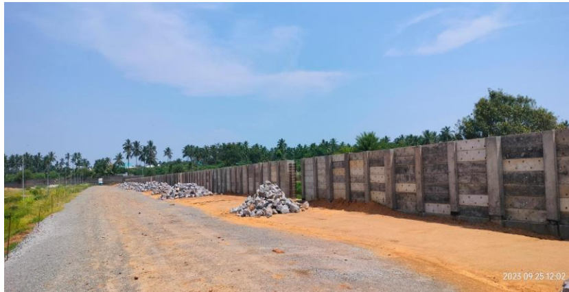
Boundary Wall & Internal Road (construction in progress)
